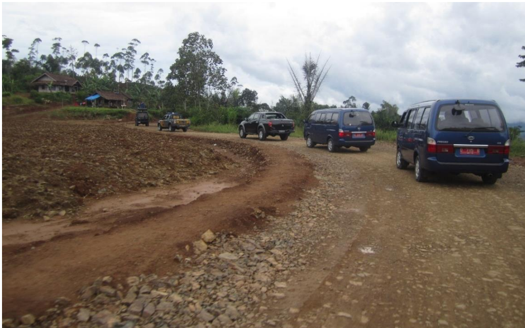
Photo 95. The vehicle group of DPRD members (DPRD West Java Province) made a working visit to carry out the function of supervising the construction of the Bandung-Pangalengan-Talegong-Cisewu-Rancabuaya vertical road, location in the Talegong area.
