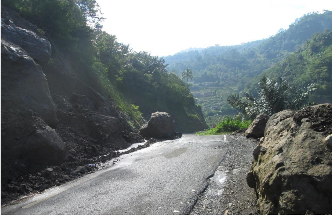
Photo 118. Landslides of rock and soil materials on roads that have been built, Talegong District.
