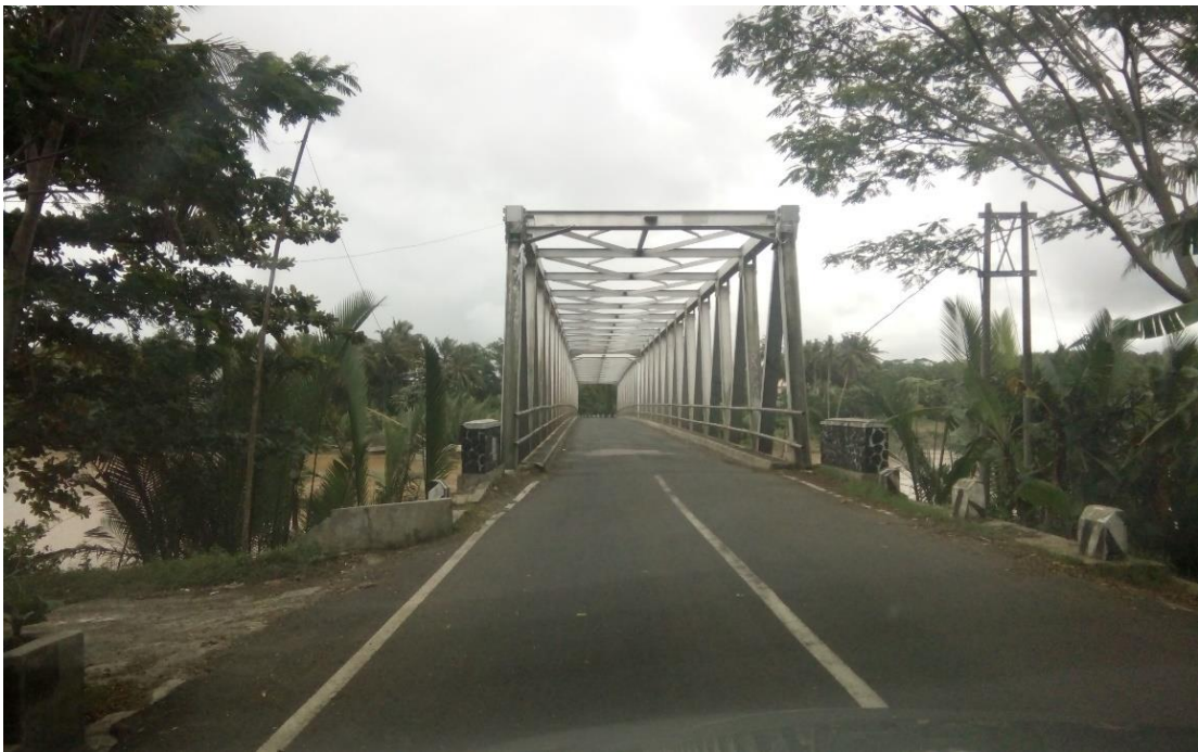
Photo 113. Horizontal Corridor of Trans SWJ Palabuanratu-Tegalbuleud-Sindangbarang-Rancabuaya-Cipatujah-Pangandaran, bridge with steel frame.
