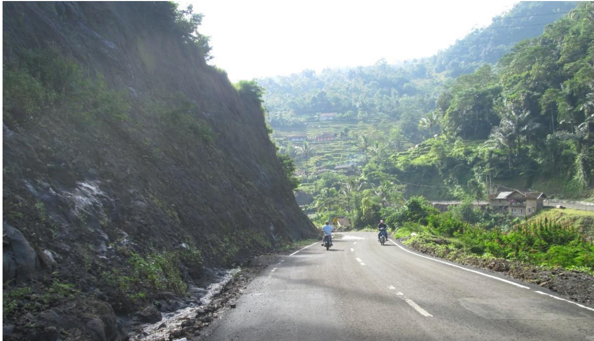
Photo 116. Steep ground contours cause landslides, Talegong District, a very sharp slope without swale.
