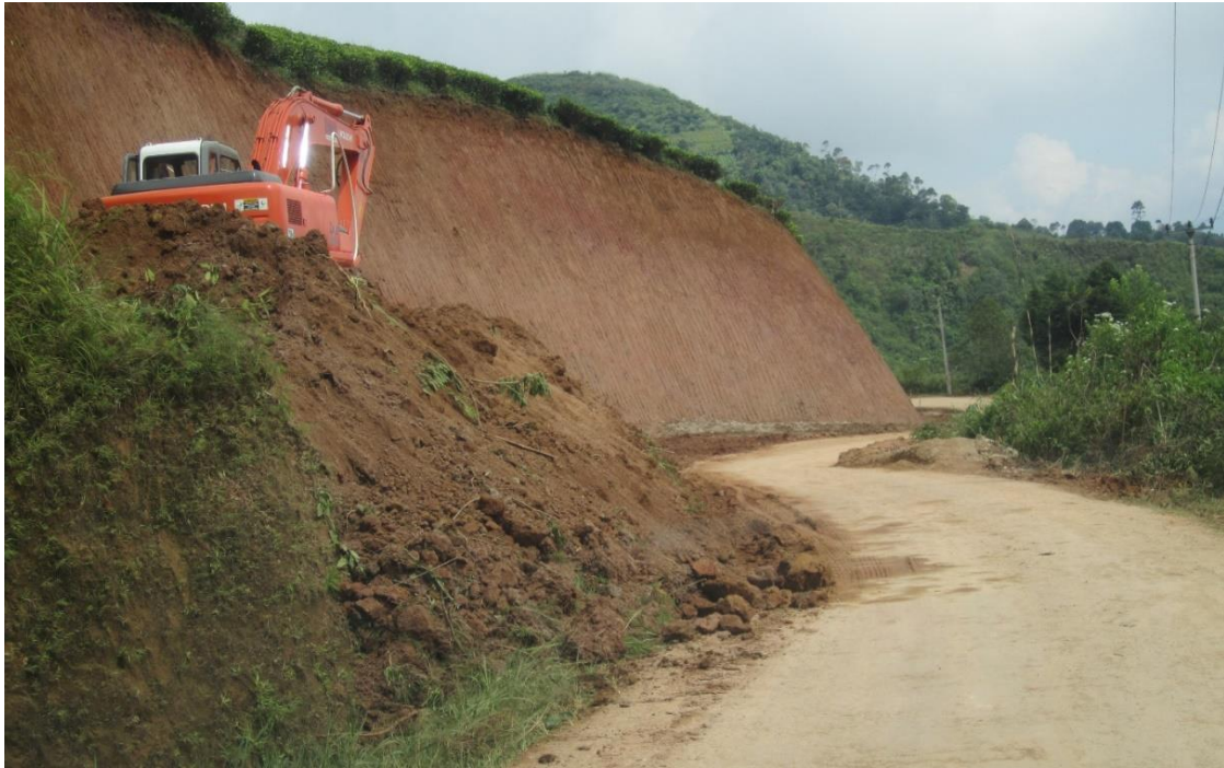
Photo 100. The Construction Process of the Bandung-Pangalengan-Talegong-Cisewu-Rancabuaya Corridor Vertical Road.
