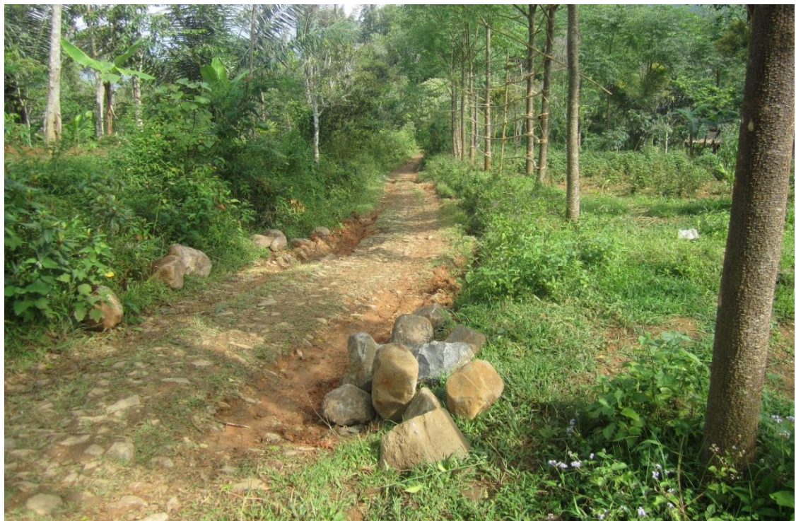
Photo 85. Puncak Hamerang-Tiwugenteng-Amlong way is very damaged and unfit.
