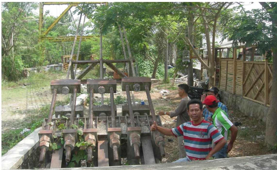
Photo 8. Cimandiri Bridge Construction (Surade District, South Sukabumi), stainless steel material.
