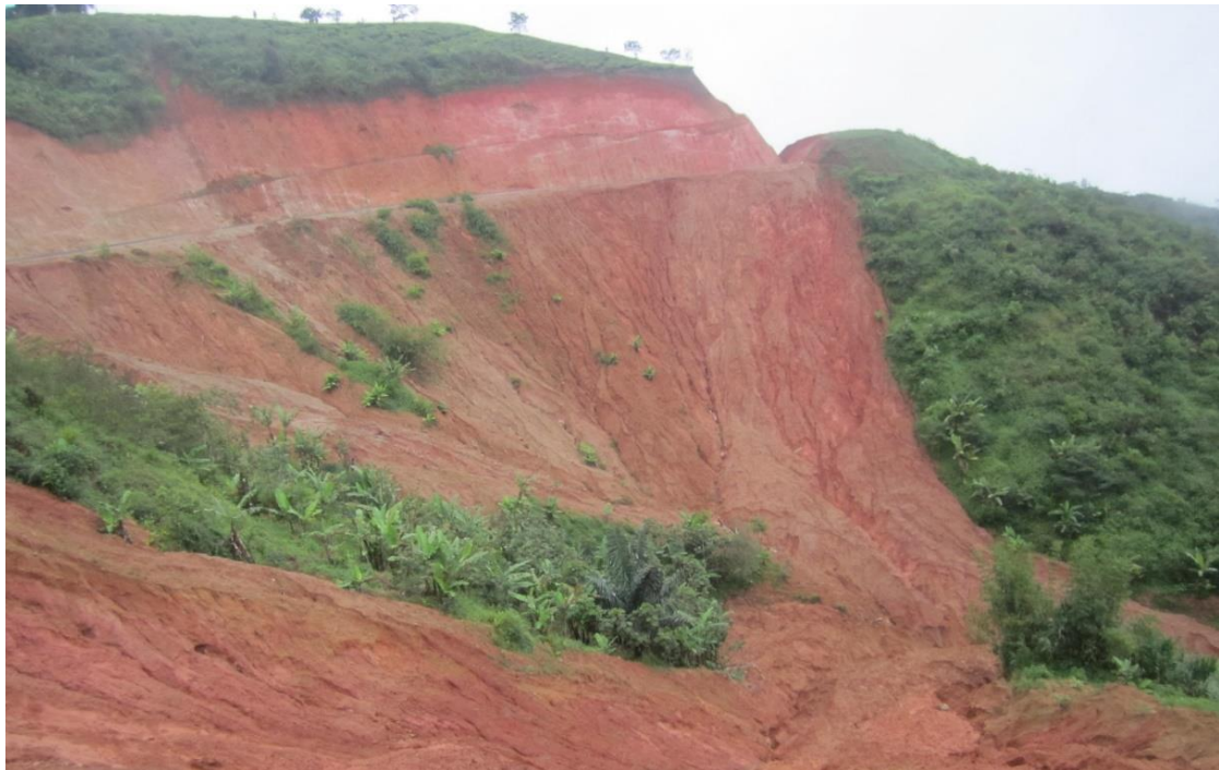
Photo 120. Landslides of soil materials on roads that have been built, Talegong District, landslide threat in the rainy season.
