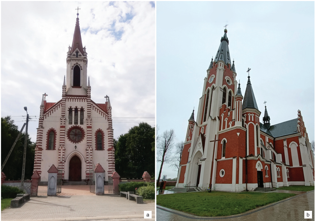
Fig. 5. Photos illustrating the decorative façade of neo-Gothic churches: a) the parish church of St. Augustine and Anthony Paderewski in Różanka, plastered on the outside, b) decorative red brick façade of St. Vitus Church in Melgwy (photo by A. Chęć-Małyszek)
