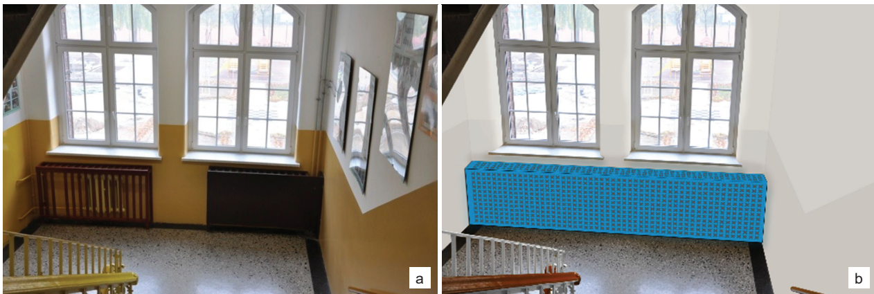
Fig. 9. Maria Dąbrowska Primary School No. 1 in Wrocław – landing between the 2 nd and 3 rd floors: a) current state, b) planned changes (elaborated and photo by E. Netczuk-Pol, 2017)
