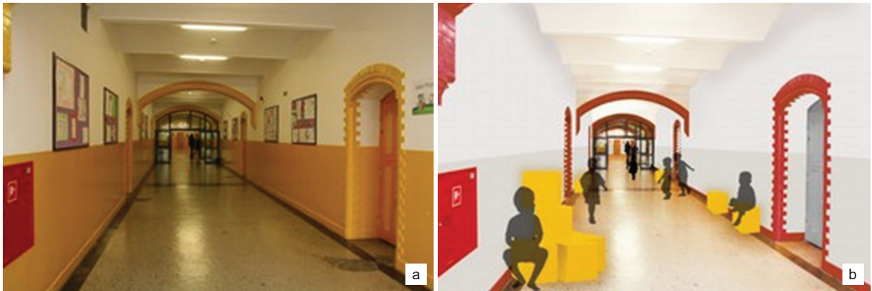
Fig. 6. Maria Dąbrowska Primary School No. 1 in Wrocław – 1 st floor: a) current state, b) planned changes (elaborated and photo by E. Netczuk-Pol, 2017)
