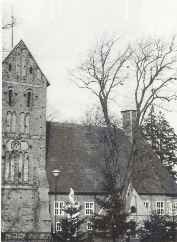
6. Krupy. Nawa z 1570 r., po 1882 r. pokryta łupkiem 6. Krupy. Nave from 1570, after 1882 covered with slate
