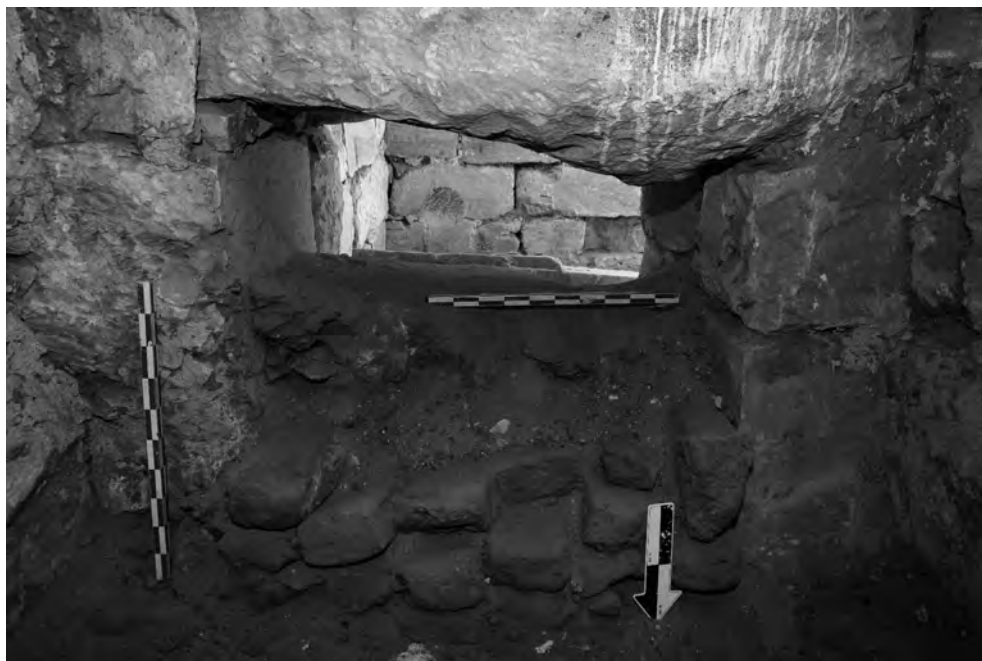
Fig. 6 The partition wall built in the entrance to the access passage leading to the burial chamber (photo J. Krejčí)
