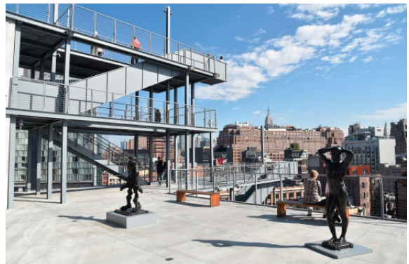
10. Outer staircases and terraces are used by the public as the main way of communication between museum galleries
