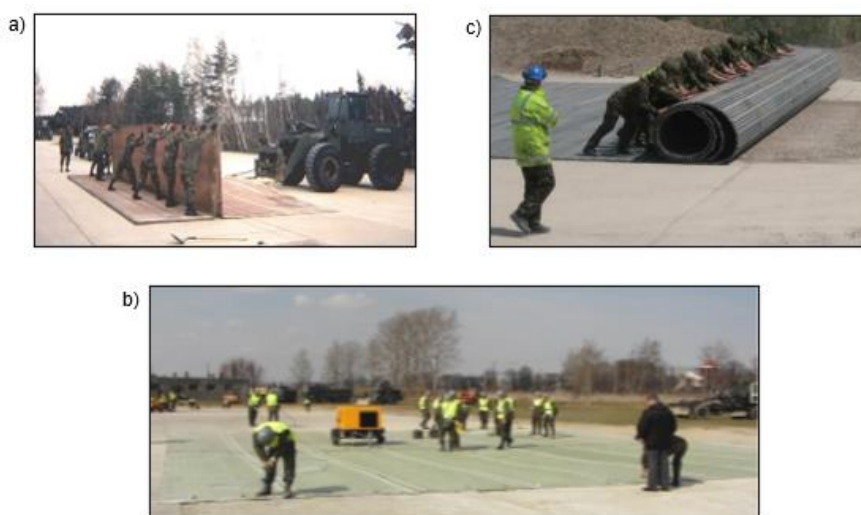
Fig. 5. Airport coverings for rapid reconstruction of airport pavements: a) FFM composite mat, b) KRATER composite mat, c) Class 60 aluminum mat, [5].
