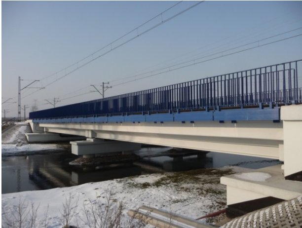
Figure 24: “Wiarna Rzeka” railway bridge in Poland, the first implementation of the clothoidal shape of dowels
