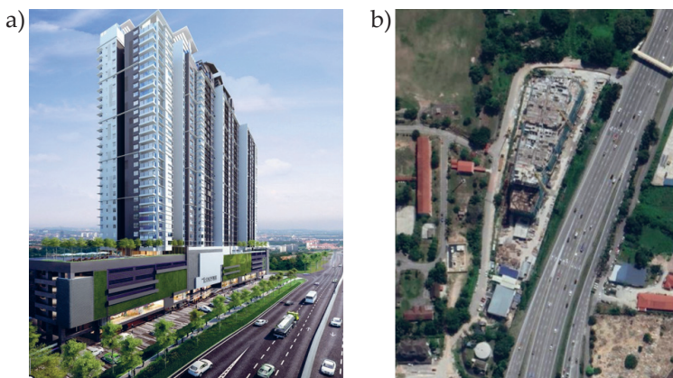
Fig. 3. High-rise building illustration (a) and satellite imagery (b)
