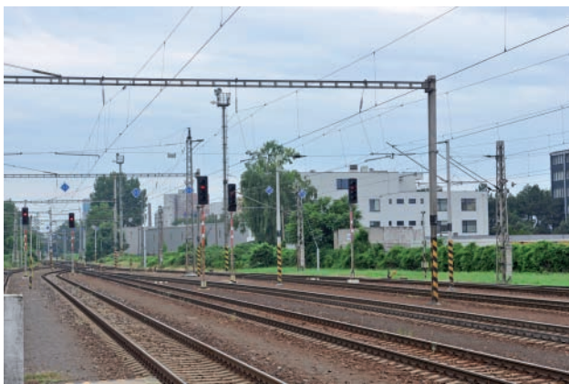
Fig. 6. Dual-voltage Bratislava Petržalka station (25 kV 50 Hz, 15 kV 16.7 Hz) (22.06.2019) [photo: M. Graff]
