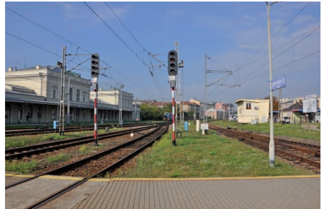
Fig. 2. Przemysł Gł. station is the border station with UZ network: on the left is the 3 kV DC electrified line LK 91 (1435 mm), on the right – the line LK 92 (1520 mm) (16.09.2016) [photo: M. Graff]
