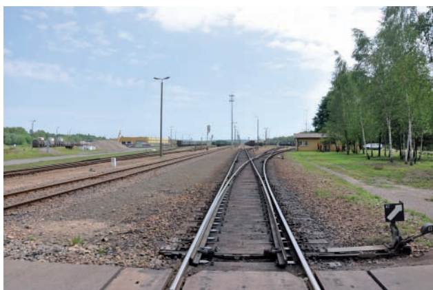
Fig. 10. The Sławków station on the LHS / LK 65 (1520 mm), western turnout point (25.06.2016) [photo: by M. Graff]
