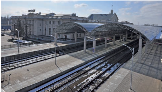
Fig. 4. Brest Central station is located at the Polish-Belarusian border and the so-called Warsaw part of the station is present: two tracks from the left with a rail gauge of 1435 mm and electrified with 3 kV DC, and two next (from the right) – wide gauge tracks (1520 mm) electrified with 25 kV 50 Hz (25.02.2018) [photo: M. Graff]
