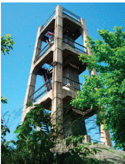
Photo 5. The observation tower before renovation
