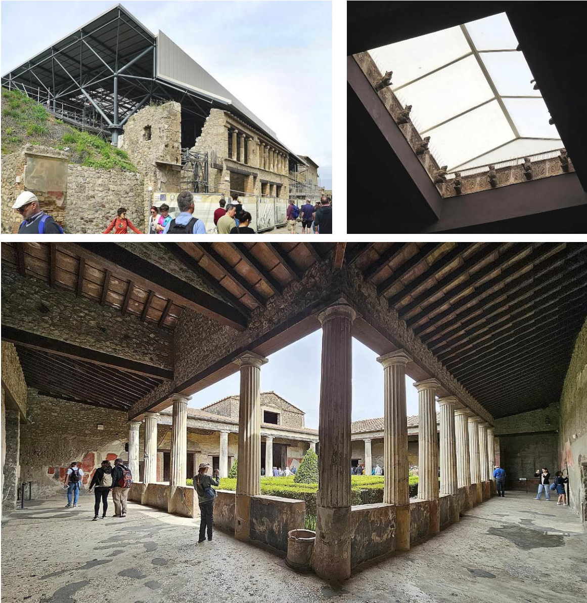
Fig. 50-52. Pompeii Archaeological Park - examples of the reconstruction of the roofs of the porticoes surrounding the atrium (bottom), the modern total roofing of the house complex (insulae), and the modern steel and glass skylight over the former atrium. Source: photo by author
