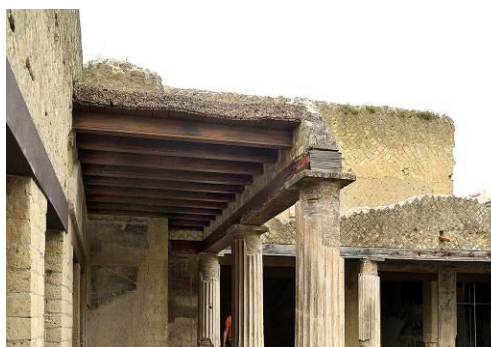
Fig. 33-35. Typical roof structures of Pompeian villas, reinforced with steel or reinforced concrete in reconstructions. Sources: Mazois 1812, photo by author
