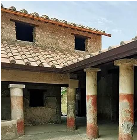
Fig. 30-32. Pompeii, an example of roof reconstruction using clay tile with "flat" tiles and covering semicircular elements. Sources: Kubicz 2021, Roman Roof 2022, Roman Tile.. 2021
