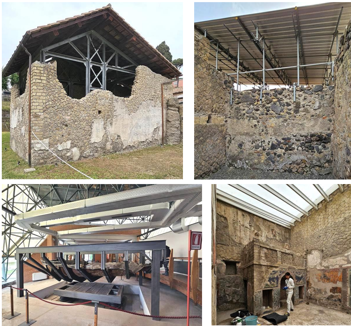
Fig. 46-49. Steel structures supporting the reconstructions in the form of roofs, roofs protecting the interiors from the influence of external conditions and supporting the exhibited artifacts - here - elements of a wooden boat (bottom left). Source: author's photo.
