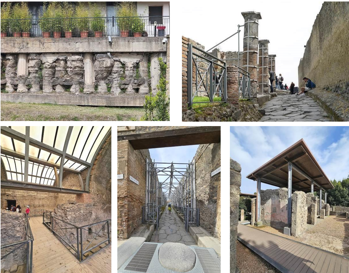
Fig. 41-45. Boscovale, Villa Regina - protection of a several-meter-long excavation wall with a reinforced concrete pile structure (top left); Pompeii Archaeological Park - examples of modern steel structures protecting and stabilizing original column and wall fragments, as well as skylights and roofs protecting walls and interiors from precipitation.
