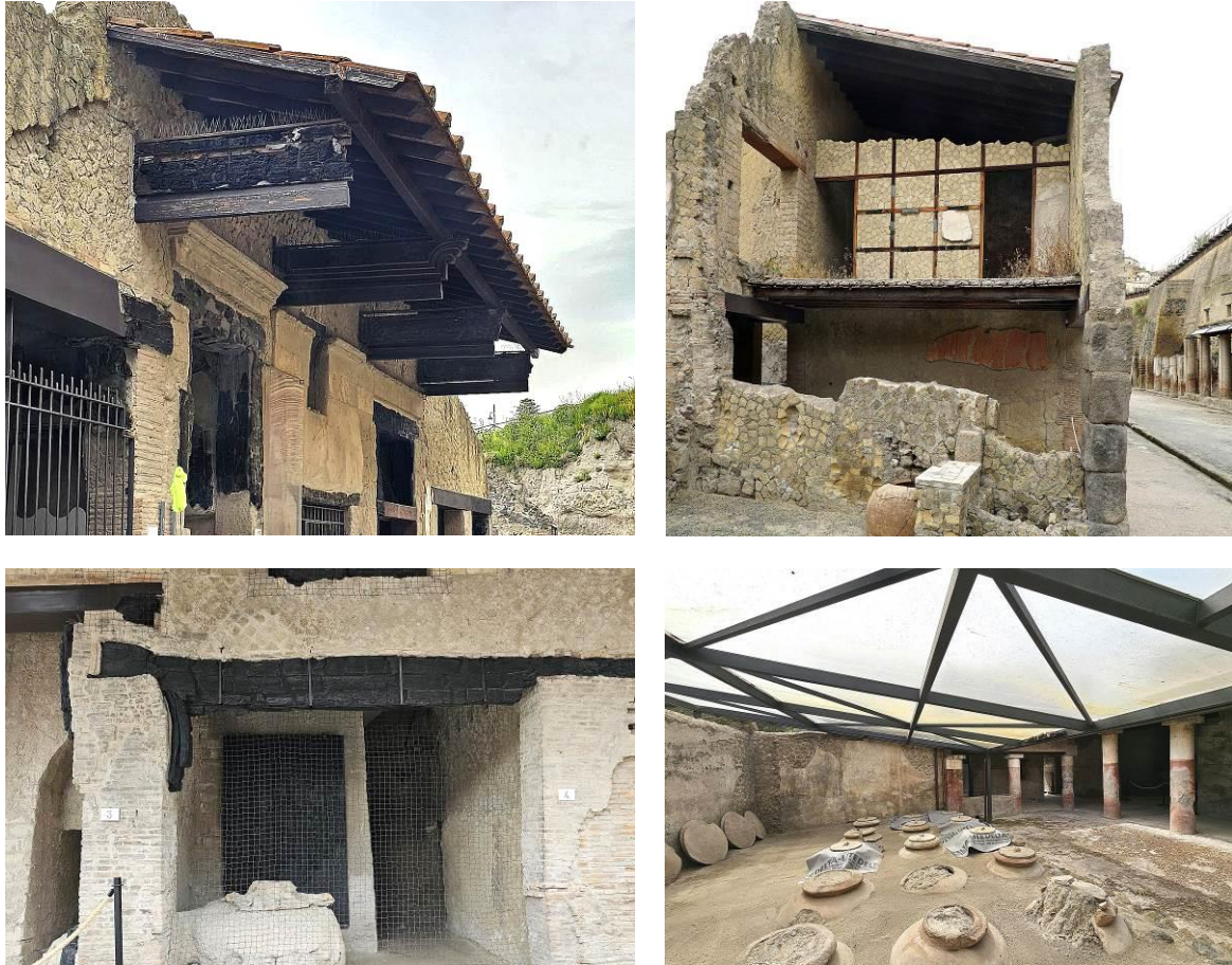
Fig. 37-40. Herculaneum - reconstructions of wooden ceiling beams, lintels and brackets showing their original charred fragments; Boscoreale, Villa Regina - a contemporary steel and glass skylight over the villa's storage room. Source: author's photo
