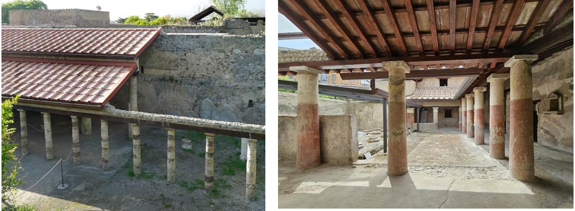
Fig. 53-54. Pompeii, a section of the reconstructed peristyle of Villa Diomedes (left) and the reconstructed peristyle of Villa Regina in Boscoreale. /source: photo by author/.
