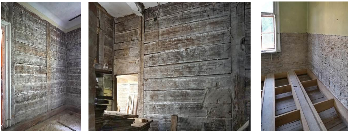
Fig. 39-41. Conservation renovation of the Rzućów manor house – the post-and-plank, larch walls of the ground floor and the walls of the ground floor (right) cleaned of their original internal plasterwork on reeds. Source: original photo 2023
