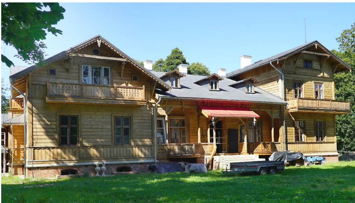
Fig. 19, 20, 21. Rzuców Manor, comparison of the state of preservation of the siding and details of the south facade – photographs from the inter-war period (top), contemporary photograph during conservation repairs. Source: photos 19, 20 – Opracowanie badawcze 2013, photo 21 – author 2023
