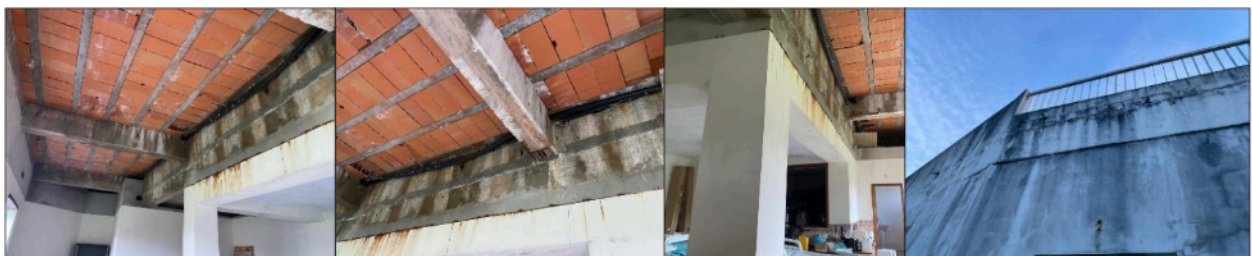
Fig. 11. Interior and exterior of the structure correspondent lines 4 and 5.
