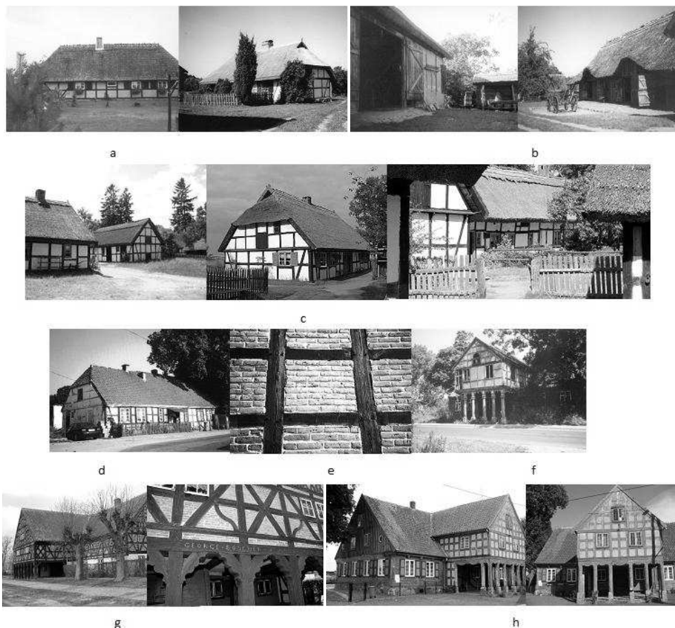
FIGURE 1. Selected examples of the ancient skeleton construction: a – Cassubian hut from 1802 rebuilt in 1984, Karwieńskie Błota; b – Cassubian hut, barn and cowshed in an antic rich farmer’s farmstead, Nadole; c – farmstead buildings, Kluki; d – dwelling house, Smolno; e – a detail of a post-and-beam wall filled with ceramic brick in a farm building from the end of the 19 th century, Darżlubie; f – canopy house from the beginning of the 19 th century, designed by a Gdańsk architect Piotr Loewen, Żuławki, Warmia; g – canopy house from 1720, Trutnowy; h – canopy house from 1840, Nowa Kościelnica (photo by Mirosława Górecka)
