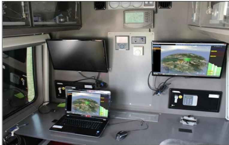
Fig. 5 Operator's compartment of the Mobile Controller Vehicle
