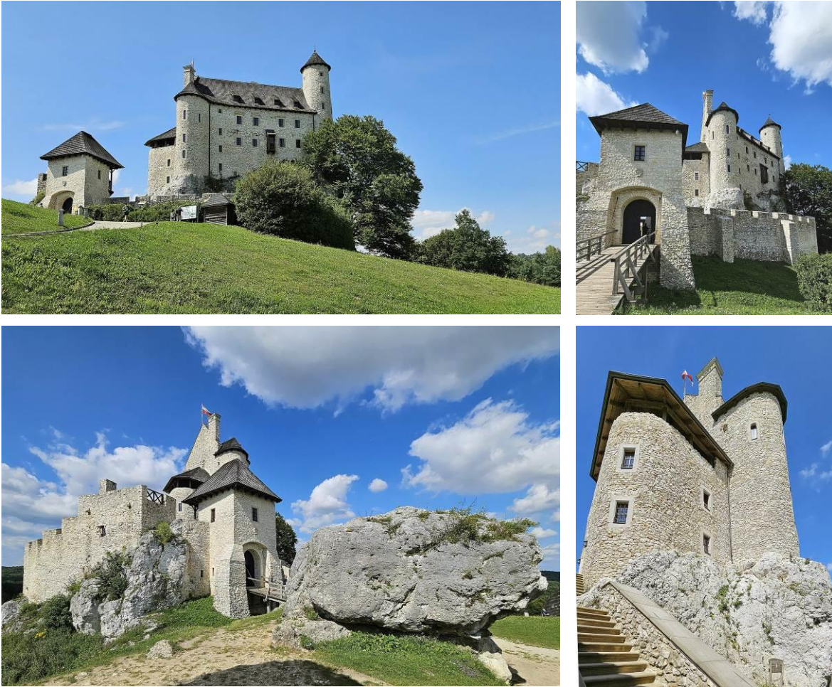
Fig. 31-34. Bobolice Castle, present state - during reconstruction work carried out on the basis of many years of archaeological and architectural research. Source: author's photo, 2024
