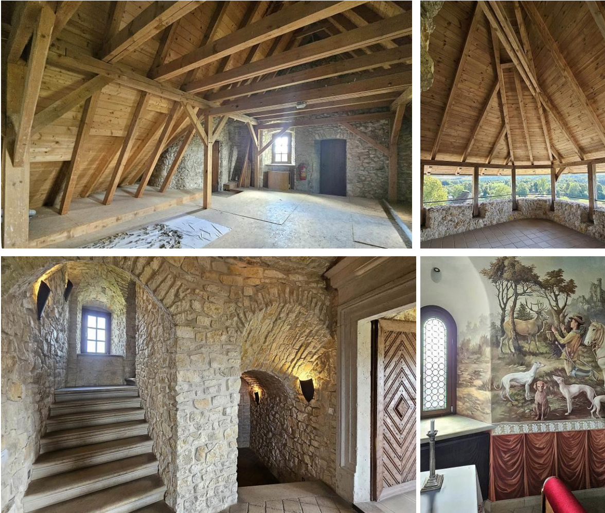
Fig. 44-47. Bobolice, castle – wooden roof structure, roofing of the observation deck, interior stairs and decoration of the castle chapel. Source: photos by author, 2024.
