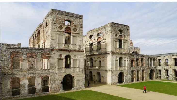
Fig. 76. Krzyżtopór Castle, the main inner courtyard and the main 4-story part of the palace. Source: photo by author, 2017
