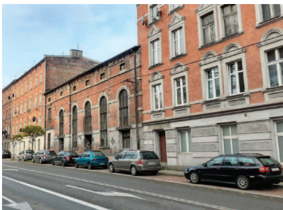
Photo 3. Current view of the adapted building in the perspective/spatial view of Styczyńskiego Street [18]
