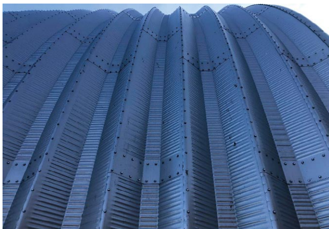
Rys. 3. Zadaszenie w systemie TG Buildings
