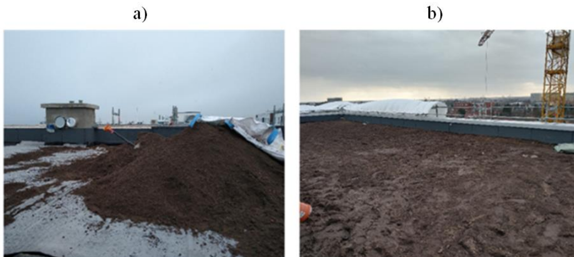
Figure 9. a) Spreading the roof substrate layer; b) Layer of roof substrate (Strzeszewska, 2023).
