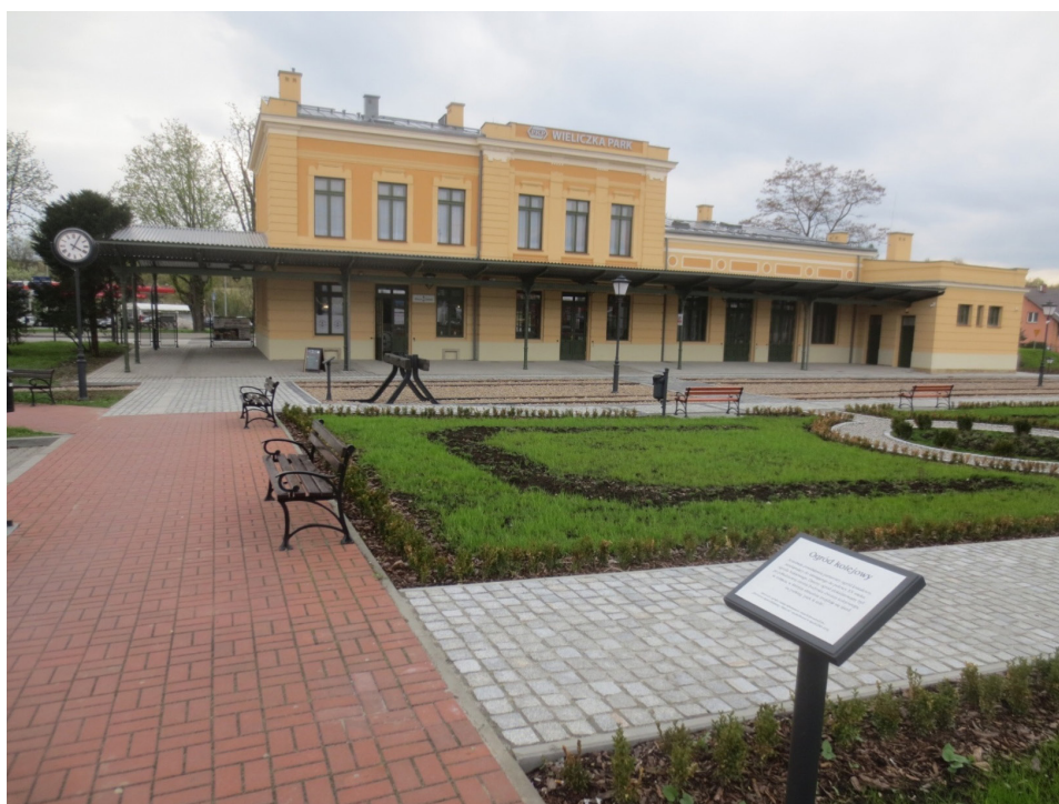
Fig. 22 Wieliczka, historic railway station building, erected around 1904, restored in 2015-2016, with a railway garden created next to it (photo: 2017)
