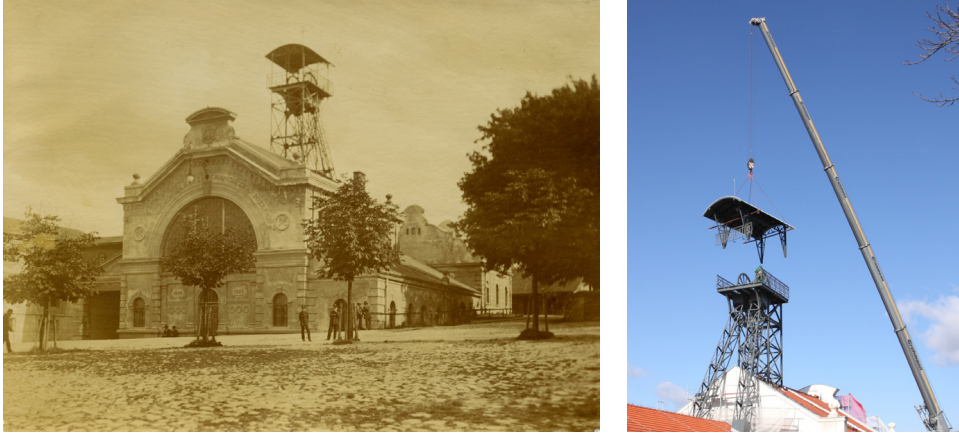
Fig. 17 Wieliczka, the steel hoist tower of the then Kaiser Franz Joseph I shaft, c. 1913 (photo from the Cracow Saltworks Museum in Wieliczka, Special Collections, inv. no. 1265/1) and its reconstruction in historical form at the present Regis shaft in 2012 (photo: J. Kucharz)
