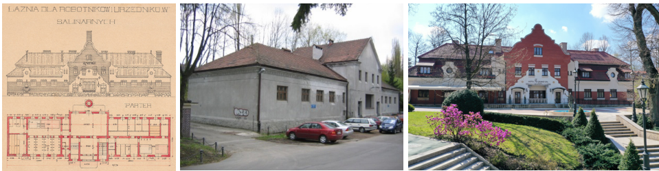
Fig. 12. Wieliczka, former bathhouse for salt mine workers and officials, drawing by K. Słotwiński, c. 1908 (Cracow Saltworks Museum Wieliczka, Cartographic Collection, inv. no. VII/2319/1, fragment), the state of the devastated building in 2005 and the state after conversion into the Grand Sal Hotel in 2009 (photo: 2021)
