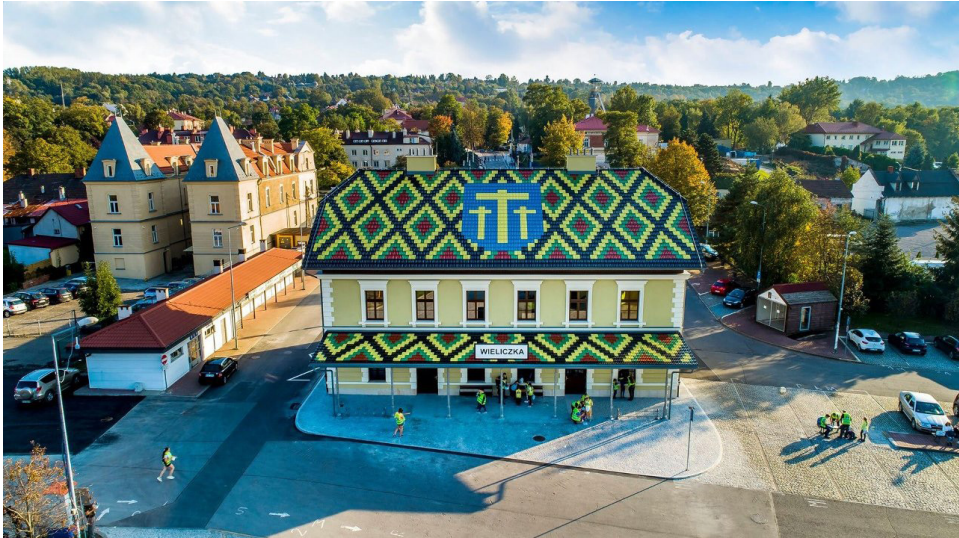
Fig. 23. Wieliczka, new public transport station, built in 2020-2021 in a form adapted to the historical urban layout, referring to local building traditions, with a jerkinhead roof covered with tiles in the green and black colours of the miner's flag and the Wieliczka coat of arms arranged with blue and yellow tiles (photo: Wieliczka Town and Commune Office, 2022, retrieved January 6, 2023, from https://www.modernizacjaroku.org.pl/pl/edition/2837/object/2900/budowa-dworca-autobusowego-w-wieliczce )
