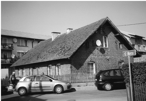
FIGURE 1. Modernization with thermal modernization of building made of red brick from the turn of 19 th and 20 th centuries. Some reservations can be expressed about the mansards of various covering forms, faced from inside with a white siding, as well as replacing the traditional ceramic roof tile with a metal one: a – state before modernization, b – state after modernization – Karwia, June 2005 – August 2008 (photo by Author)
