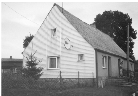
FIGURE 2. Clay dwelling house from the end of 19 th century. Only the western wall of the building is protected against wind and rain and only with siding, without insulation. Also the wooden windows had been changed to the new, plastic – Minkowice, July 2002 (photo by Author)
