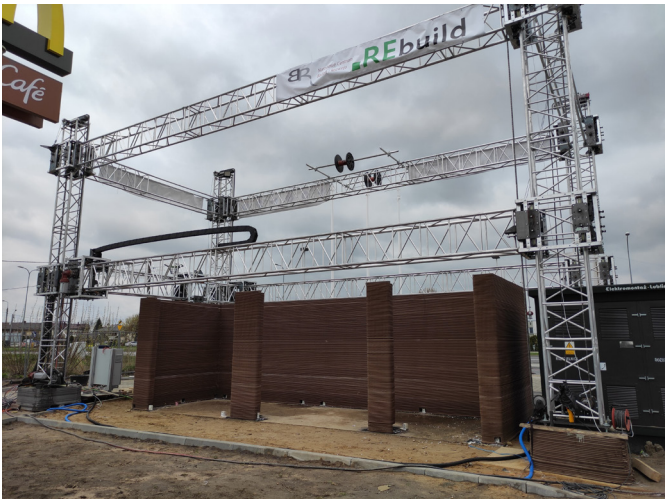
Fig. 2. Printer Rebuild v3. Real view from the first building site of this type in Poland, with the application of concrete in 3D printing
