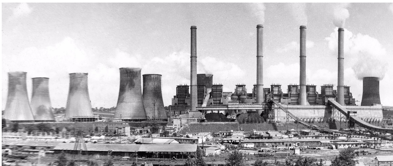
Fig. 7. 1970s - development of electricity networks - Bełchatów CHP plant
