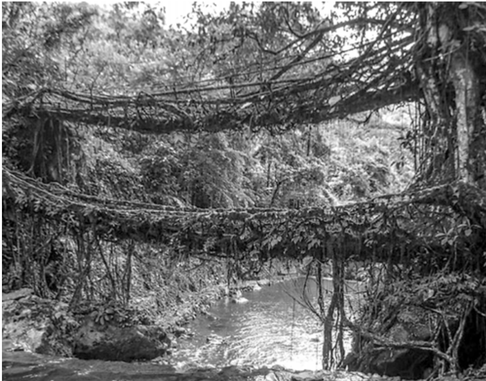
7. The construction of living root bridge completed with stones. Source: http://humanplanet.com/timothyallen/2011/03/living-root-bridges-bbc-human-planet/
