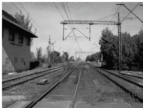
Fig. 1. Railway crossing in Krzesiny Street in Poznań, state as in August 2011; a – view in the south-western direction (direction into the military airfield), b – view in the north-eastern direction, c – condition of the pavement at the railway crossing, d – view of the railway line to Poznań Główny.
