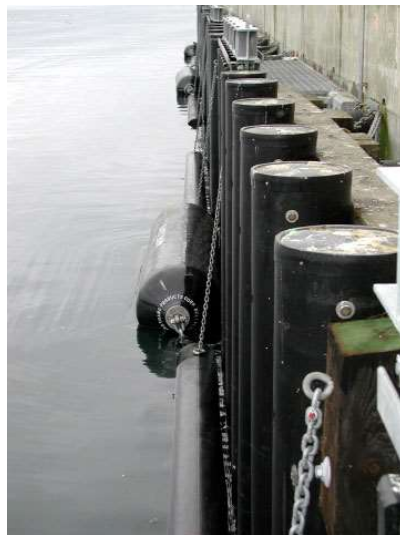
Fig. 3. Close-up of CFFT piles of the structure shown in Fig. 2 [9]
