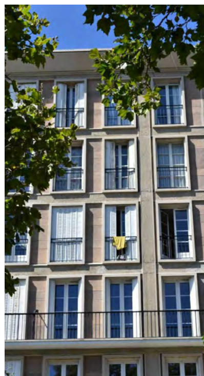
Fig. 6. Facade of a residential building, photo by Szumigata K.O., 2019
