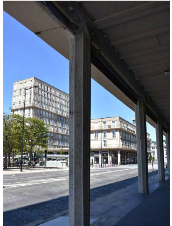
Fig. 12. Detail – play of structures on the ground floor column of a residential building in the Port West Estate, photo by Szumigala K.O., 2019
