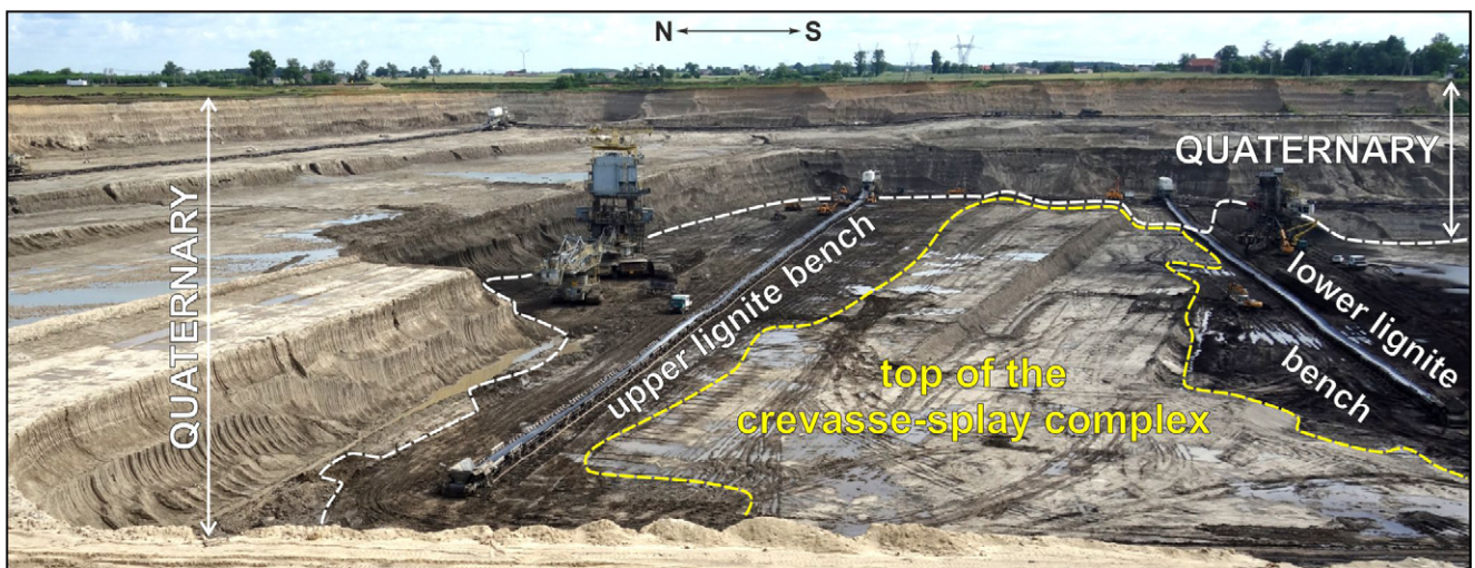
Fig. 3. Broad eastward view, showing the outcropping top of the examined sandy complex within the First Mid-Polish Lignite Seam (MPLS-1).
