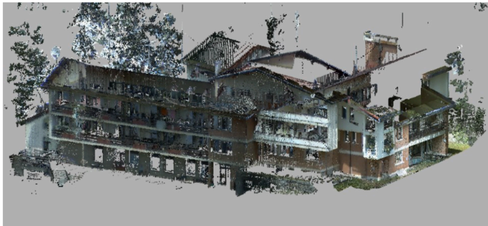
Fig. 9. Point cloud obtained by terrestrial laser scanning
