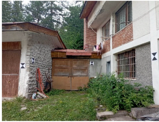
Fig. 5. Placed paper marks on the façades of the object
