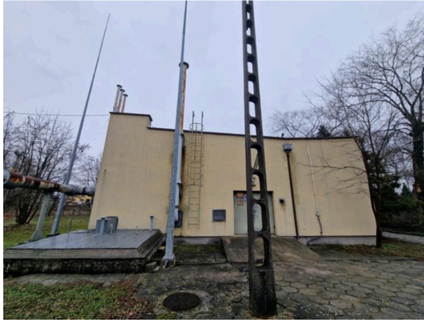
Fig. 1. The building of the methane drainage station
