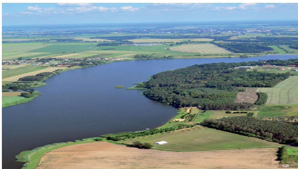
FIGURE 2. Retention reservoir Radzyny
