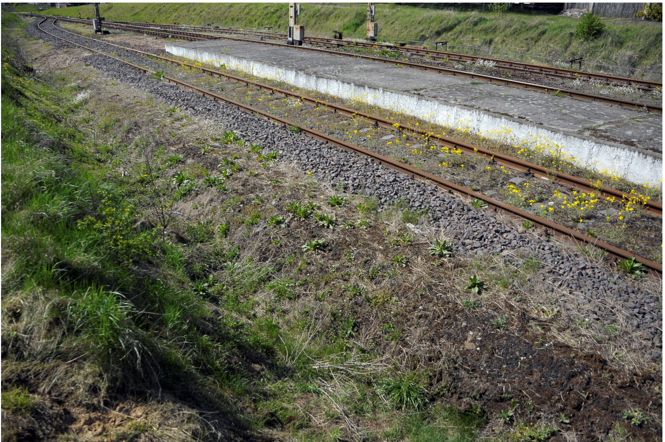
Fig 2. Site 1, railway embankment. Photo: M. FRASUNKIEWICZ
