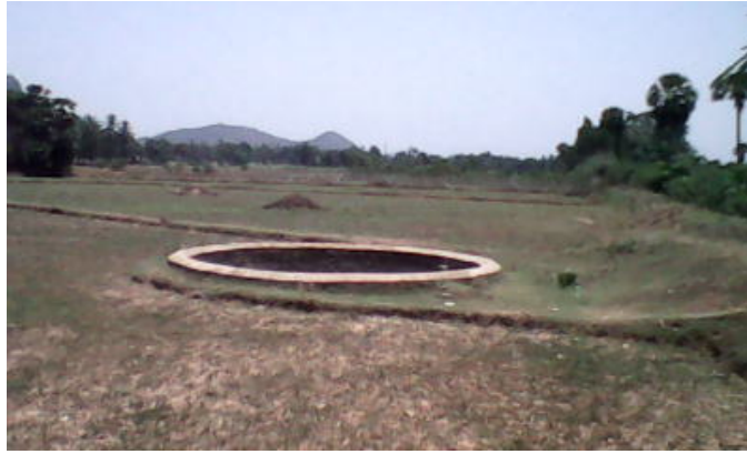
Plate 1: Open well of 6m diameter with 5.2m (bgl)water level used for agriculture along the road connecting Venkanna Palem and Murdhurty in the study area.
