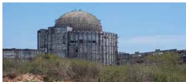
Fot. 7. Widok na 1 blok EJ Juragua na Kubie (porzucona budowa) Photo 7. A view of the Juragua NPP 1 st unit on Cuba (abandoned construction); http://www.thebohemianblog.com/2014/08/cuba-abandoned-unfinished-soviet-nuclear-power-station.html
