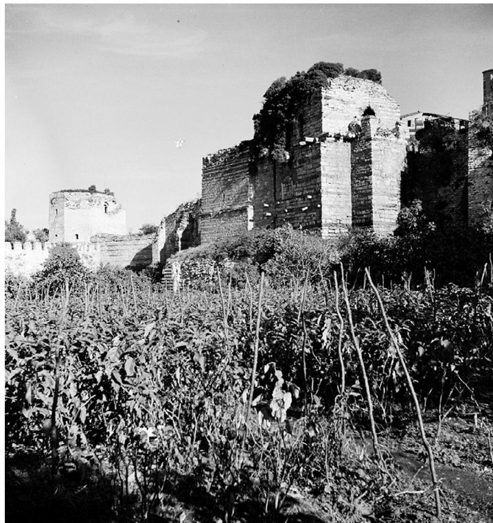
Figure 7. The tower of Isaac Angelos and the lower section of the Blachernae walls from the southwest. Market garden, possibly planted with eggplants. Source. N. V. Artamonoff, 1936, photograph, Image Collections and Fieldwork Archives, Dumbarton Oaks, Trustees for Harvard University, Washington, D.C. Licensed under CC BY-NC-SA 3.0 IGO.
