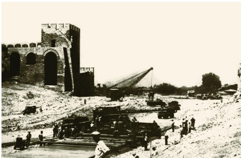
Figure 4. The concrete mixer pouring 25 cm thick concrete at the beginning of Millet Caddesi between Towers 60 and 61. Source. Unknown author, photograph, from Gül, M.: Urban planning operations and their background in Menderes period in Istanbul. In History of Istanbul from Antiquity to 21st Century , vol. 9 [online]. www.istanbultarihi.ist , 2000 [retrieved 04.05.2023, 12:20 CET]. Accessed at www.istanbultarihi.ist/715-urban-planning-operations-and-their-background-in-menderes-period-istanbul .
