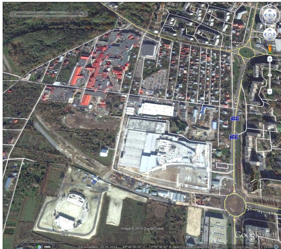
Fig. 2. Commercial-Production Complex 'Rynok Pivdenny'. Source: Google Earth
