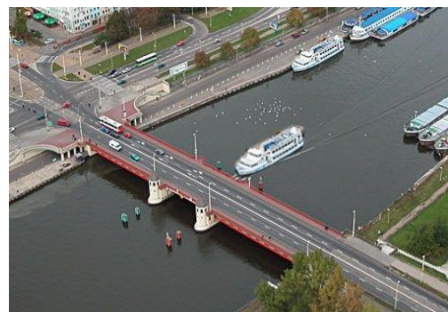
Figure 28. Dlugi Bridge in Szczecin
