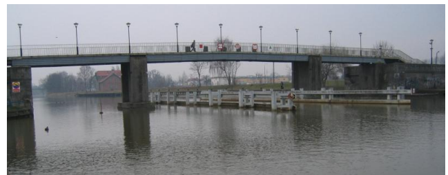
Figure 24. Lower bridge in Elblag
