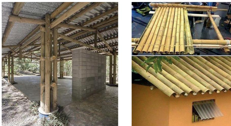
**Figure 3.** Use of bamboo culm (a) full bamboo culm as structural elements, (b) half/full culm as roofing
