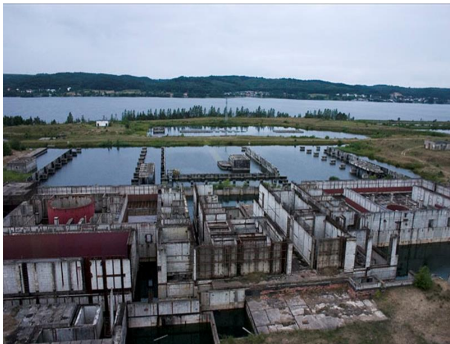
Fig. 2. Building site of the Żarnowiec Nuclear Power Plant
