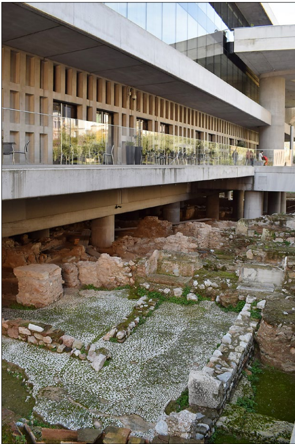
Fig. 2. New Acropolis Museum, a new idea of suspending the building above the archaeological site at the foot of the Acropolis; photo by K. Stala.
