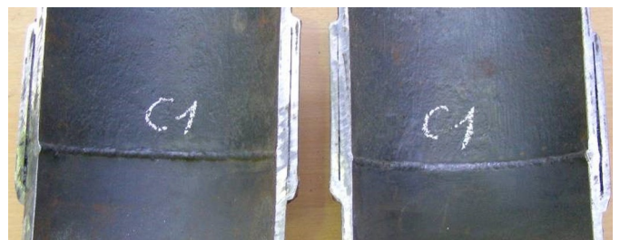
Fig. 8. View of C1 welded joint from the root side; visible sealing band
