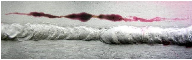
Fig. 6. View of the A1 welded joint from the root side after penetrant testing
