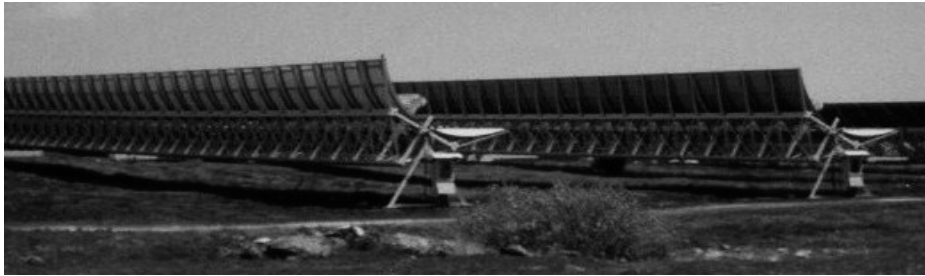
Fig. 5. View of cylindrical (pipe) concentrator of solar radiation operating at Instituto Tecnológico y de Energias Renovables (ITER) on Tenerife. Photo: Grażyna Frydrychowicz-Jastrzębska
