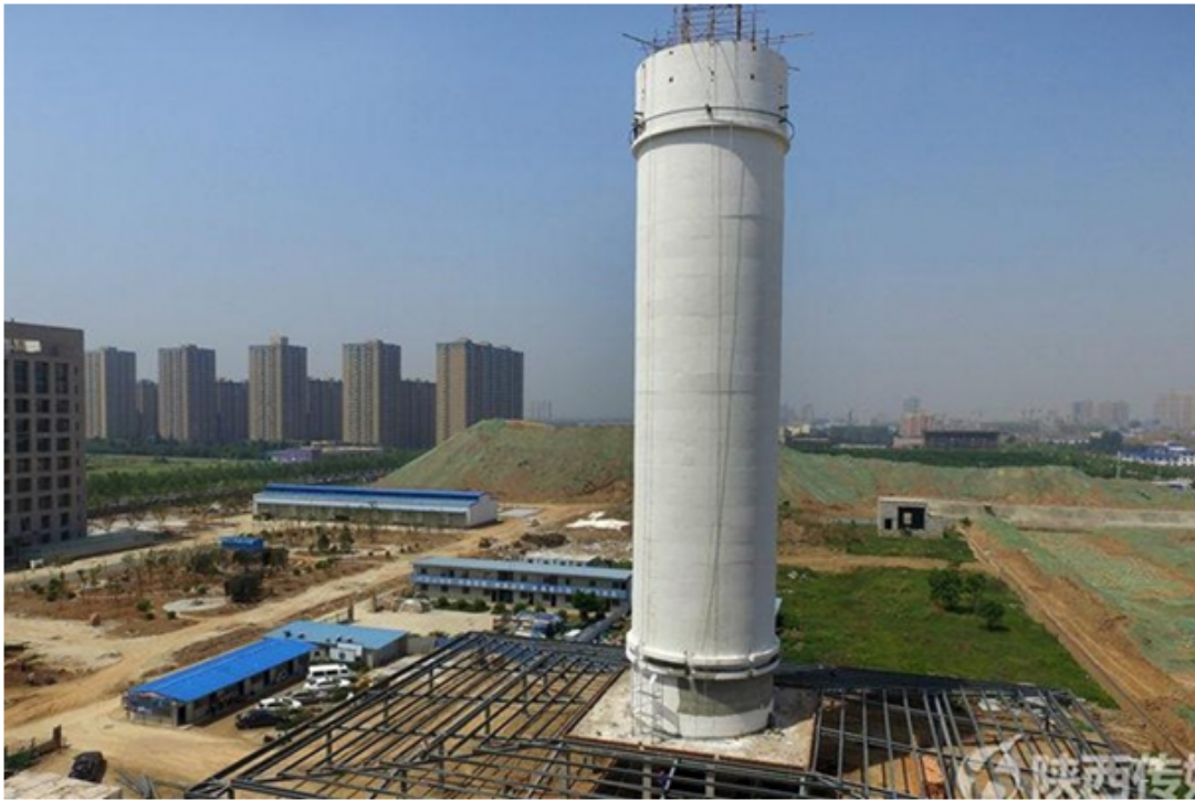
Figure 4. Air purifying tower in Xian, China [4]
