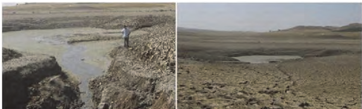
Phot. 2. The leakage of Hammam Grouz dam in 2003 (photo M. Boussekine)
