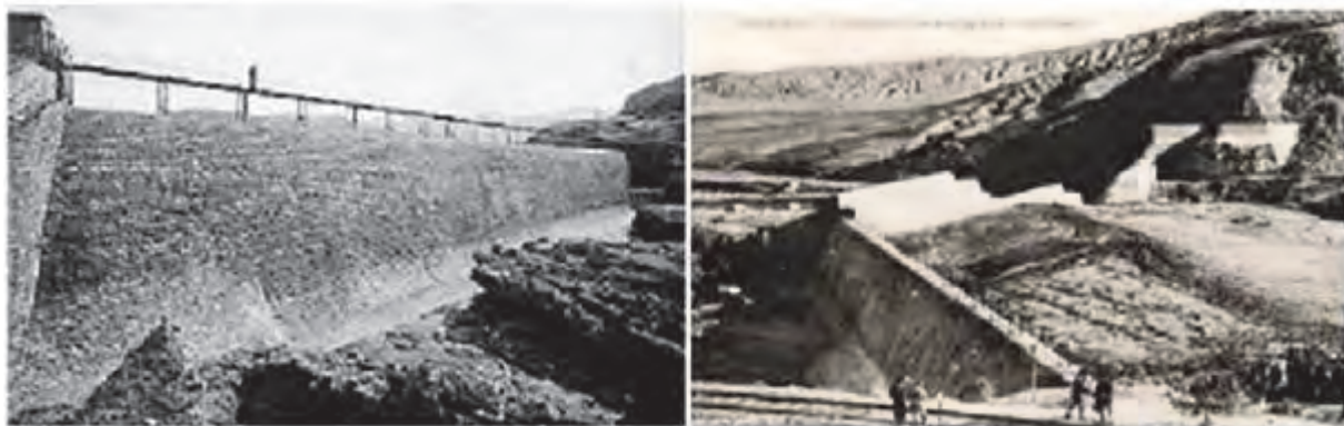
Phot. 1. Dam failure of Fergoug [BOUHLALI 2006]
