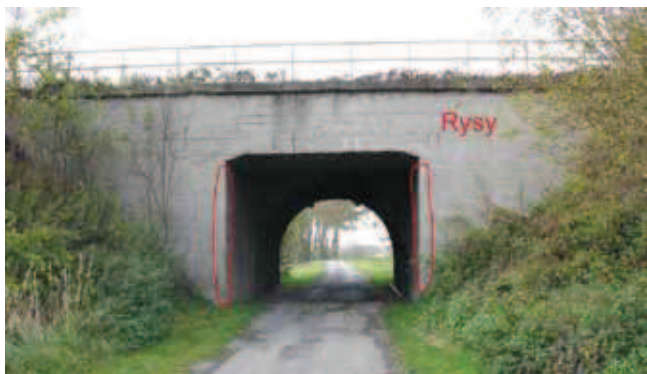
Rys. 5. Wiadukt żelbetowy (pod torem nr 2) [9] Fig. 5. Concrete viaduct (under railway track no. 2) [9]
