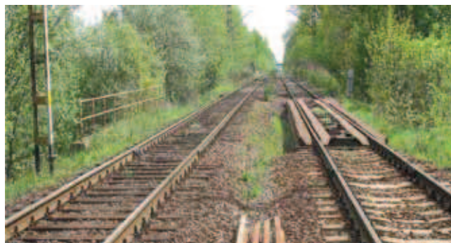
Rys. 2. Widok na tor na wiadukcie [9] Fig. 2. View on the railway track on viaduct [9]
