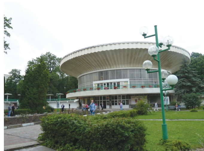
Il. 7. Morshyn. Pump room. Source: author's own materials Il. 8. Stebnyk. Derricks for coal mining. Source: author's own materials
