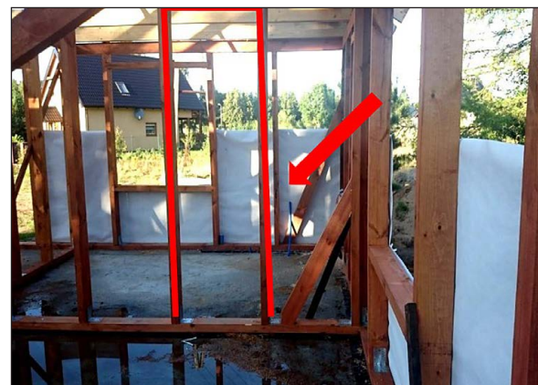
Fig. 3. Wall plane example in real wooden house
