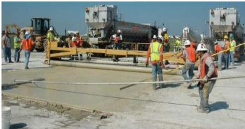
Fig. 1. Concrete works at Seattle-Tacoma Airport using a Rapid Set® mix [7]
