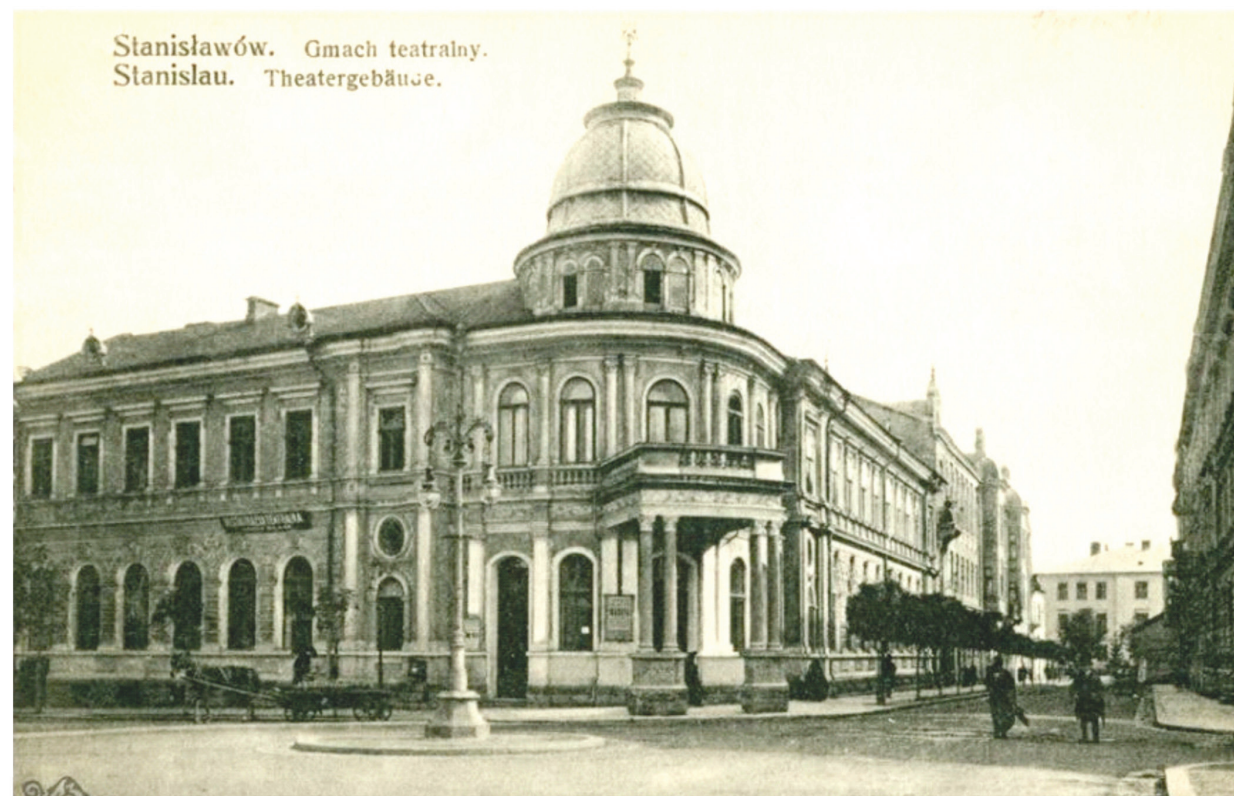
Ill. 5. Theater named after O. Fredro in Ivano-Frankivsk: a) a general view; b) a theater plan; c) the plan of the balcony [23]
